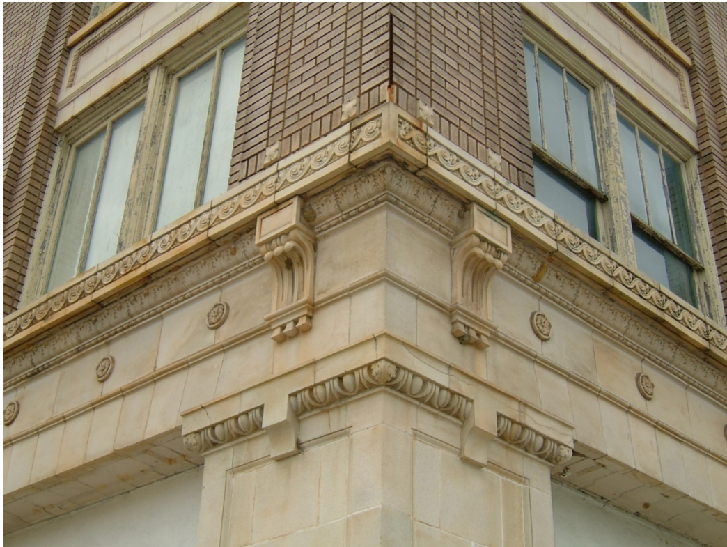
Exterior is decorative pressed brick, the interior is ornamental plaster, making the building virtually fireproof
