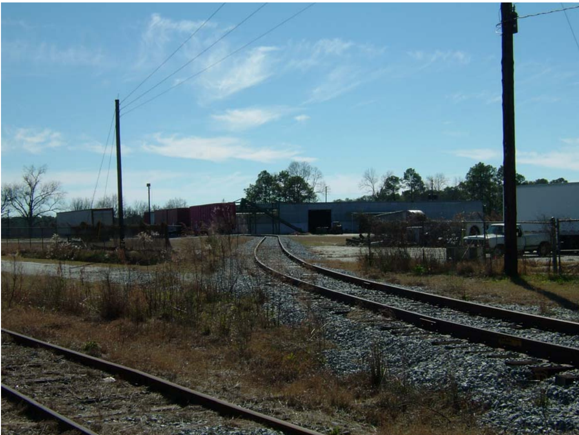
Rail spur, north side of building
