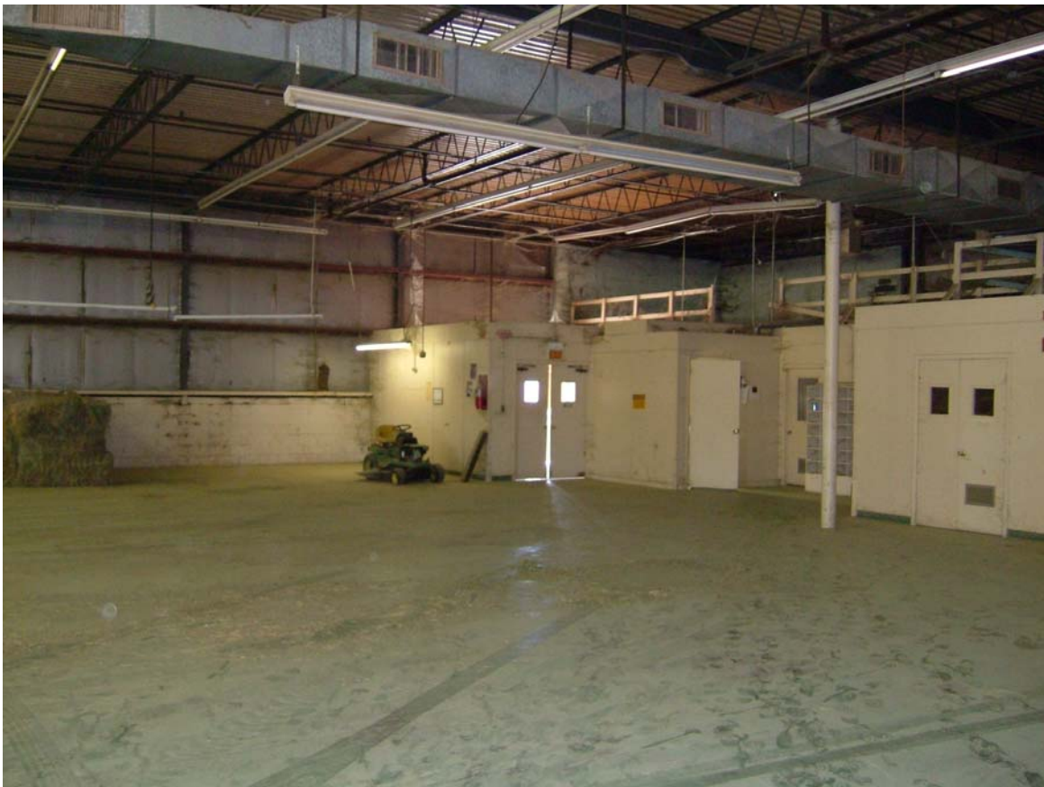
Facing office and front of building (South)
