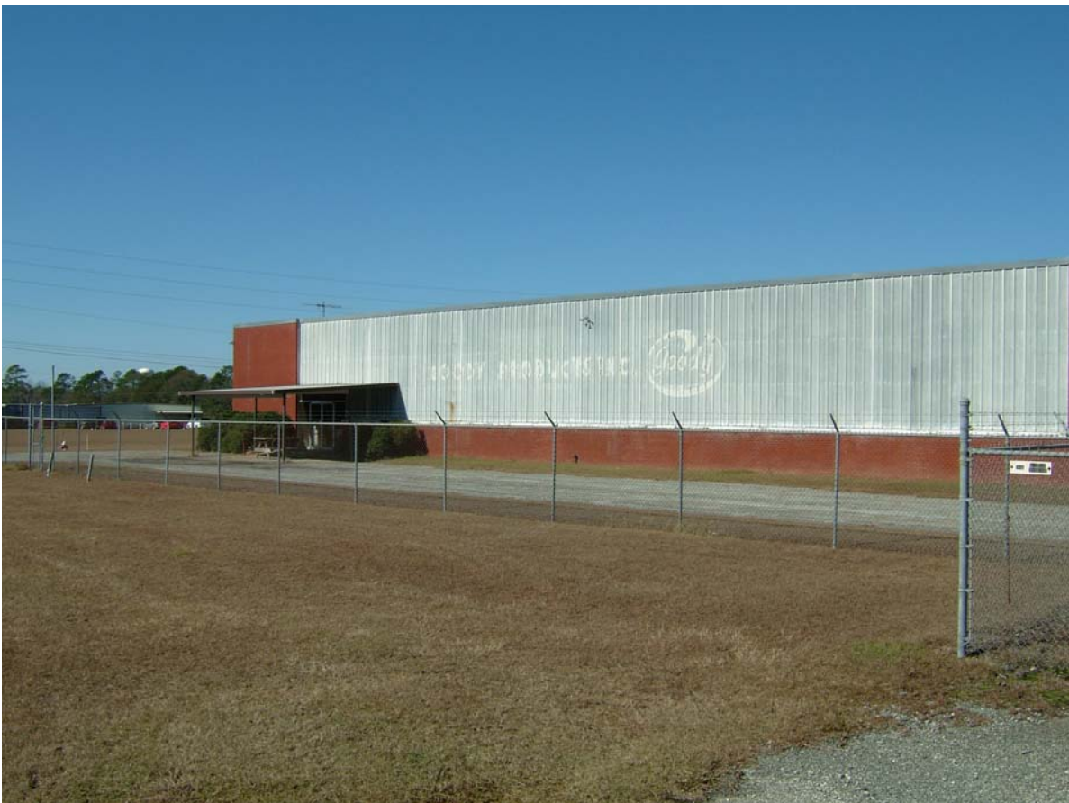
Front (south) of building
